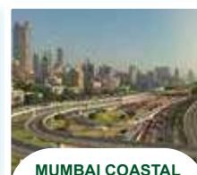
MUMBAI COASTAL ROAD MEGA PROJECT
