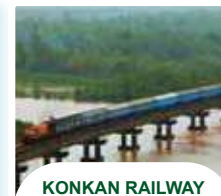
KONKAN RAILWAY PROJECT
