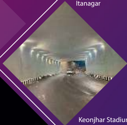
Tunnel lighting, Itanagar
